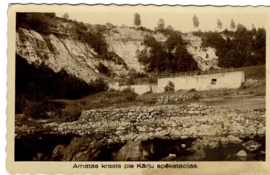
Fig. 2. Hydroelectric power plant 'Kārļi' (photo from www.zudusilatvija.lv ).
